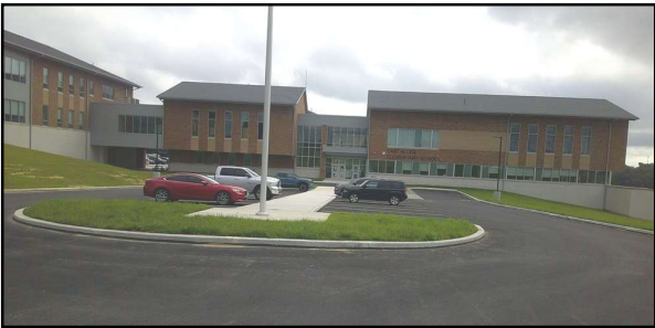
Main entrance of the East Allen Elementary School facing New Seemsville Rd. Administration and technology offices are on the left side of building. Photos by Barb Wiemann
