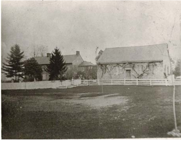
Ralston McKeen House on left, Wolf Academy on right as viewed from the west side. Note the frame addition on the south end of the RMH which was removed.
